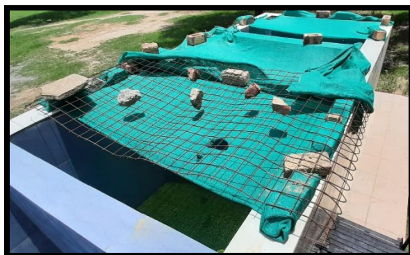
Figure 3: Cemented water tanks with net cover
